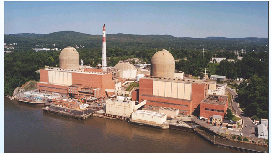
Indian Point Nuclear Power Plant
